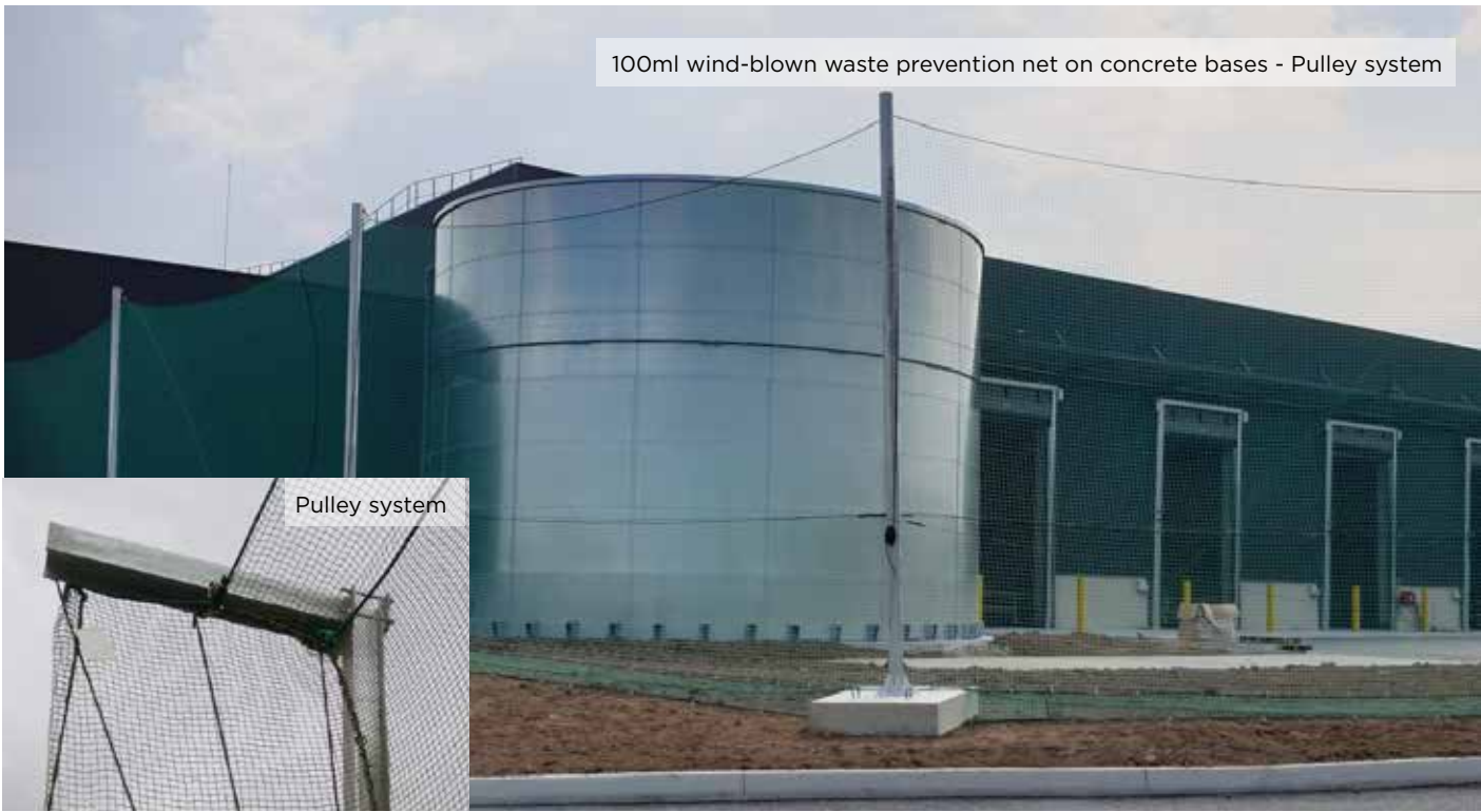
Fixed wind-blown waste prevention structure on storage bay - height 3 m
